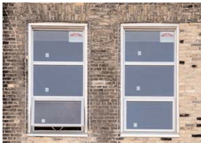
The window systems feature AFG's Ti-R low e Argon filled windows with Super Spacer high performance glass
