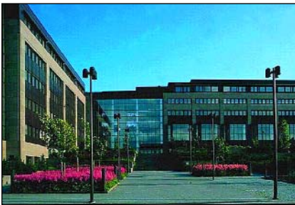
Offices of Fortum Energy Production Company Vantaa, Finland
