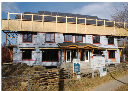
A Riverdale net zero home after the Duxton Window installation.
